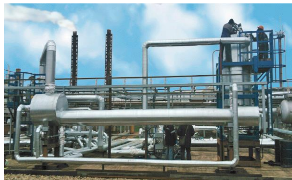
Reactor with fixed bed of catalyst
